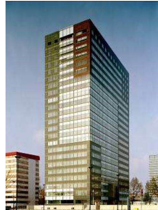
Winston Churchill Tower - Rijswijk: Renovation with a double skin facade (internally ventilated)
